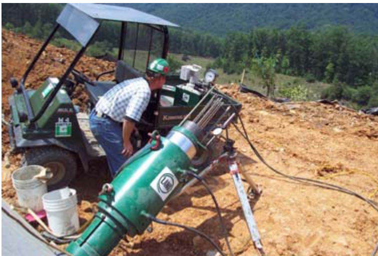
Proof loading an installed ground anchor.
